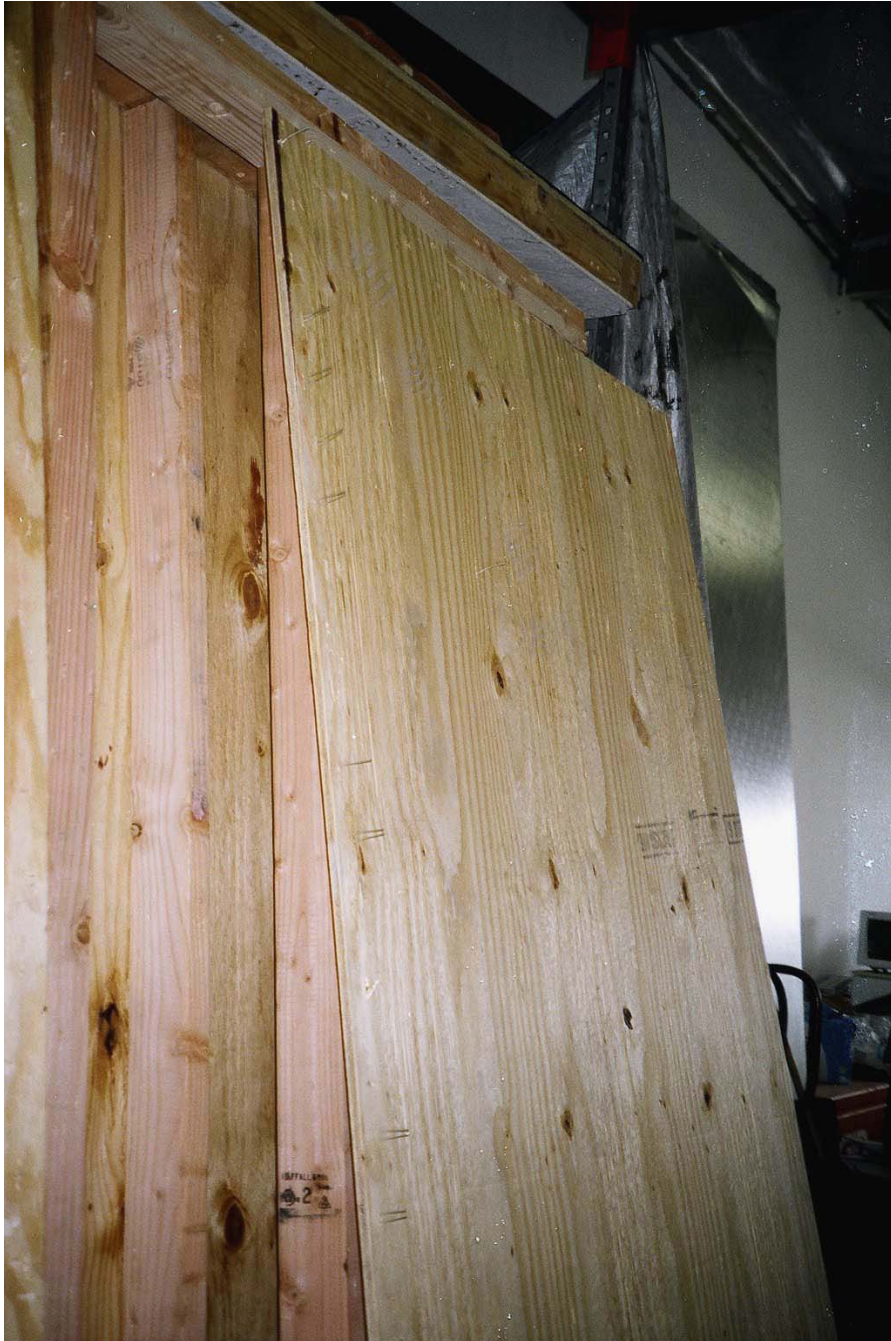
Photo 3: View of right edge of right panel, removed to show back side, with 8 staples that were still attached to the frame. No other staple legs were visible.
